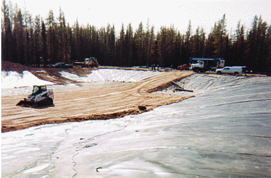
**Backfill protects liners from environmental and mechanical damage. Backfill can also help to improve the impermeability of the liner system.**
